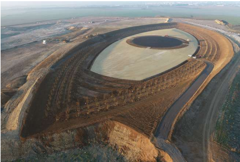
Lacil du ciel, photograph taken during realization, March 2023, Villeneuve-sous-Dammartin, France © ECT
